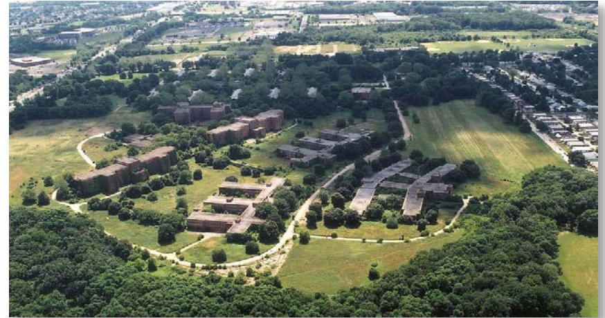
Philadelphia State Hospital at Byberry
